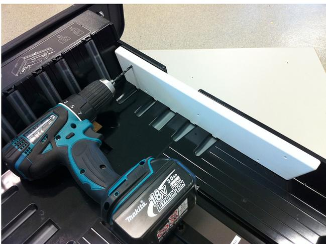
10. Place the guides in position. Drill through the two TOP holes using a 4mm speed drill.
